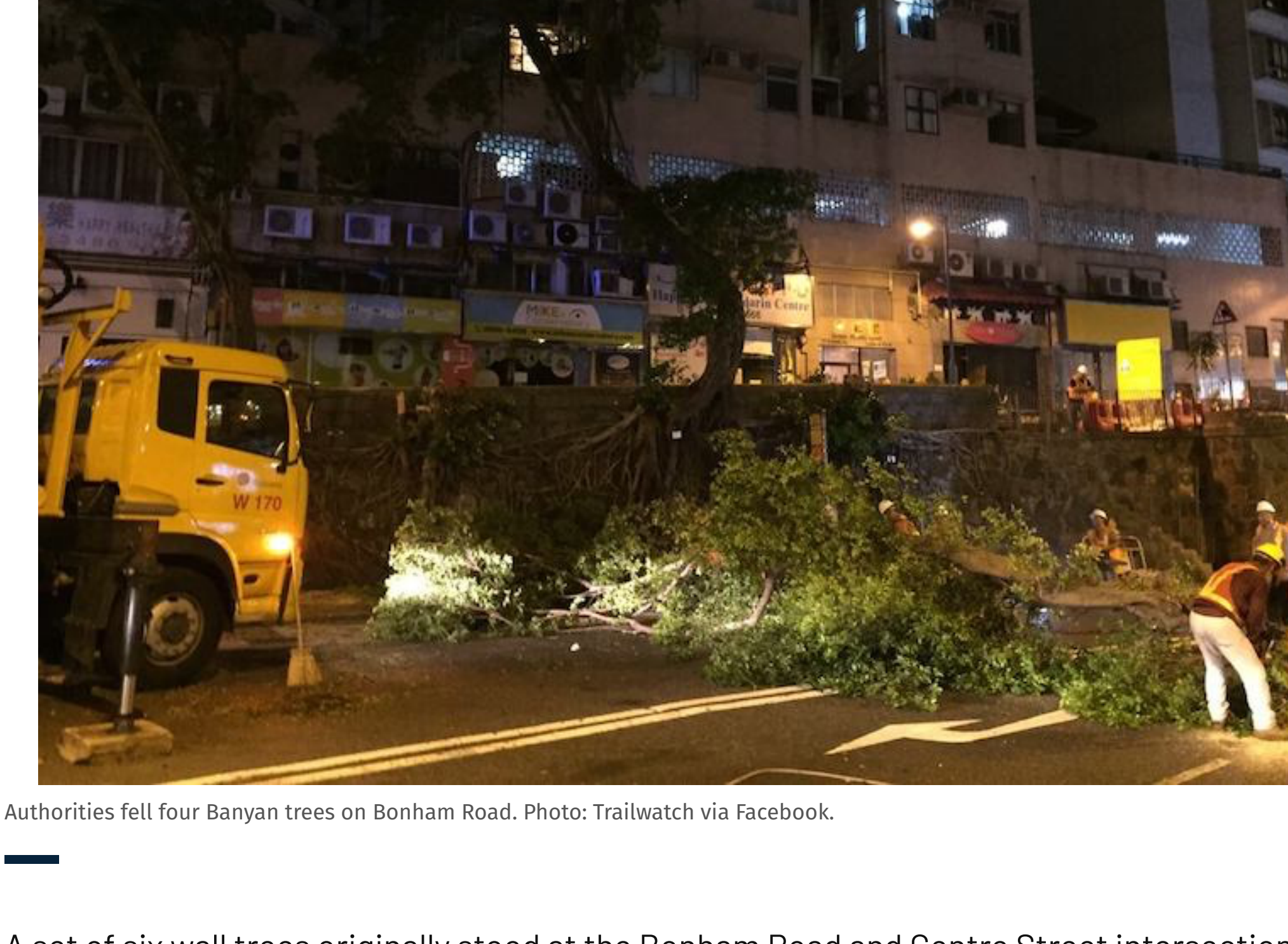
Authorities fell four Banyan trees on Bonham Road. Photo: Trailwatch via Facebook.
